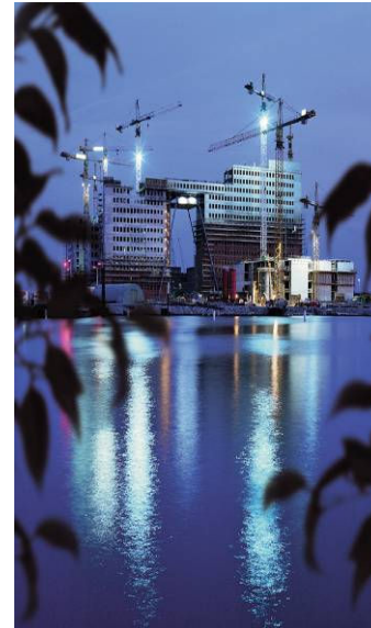
TNO Built Environment and Geosciences
